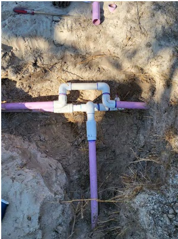
Zone pipe repair in Story Brook Park.
